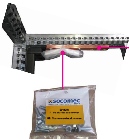
5. 10.2. Connections if the MAINS and AUX MAINS are connected IN COMMON
