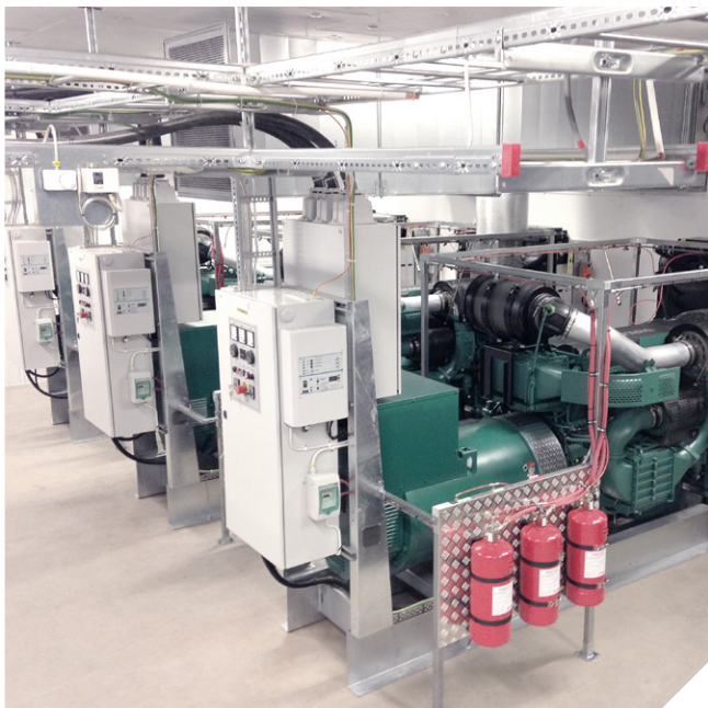
Stationary-installed emergency power system
